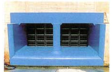
Example of an intake structure
