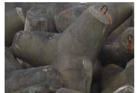
Example of tetrapod structures
