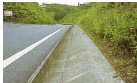
Slope side ditch at Yanbaru
